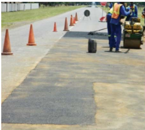
Pothole Patching – Outsourced maintenance
