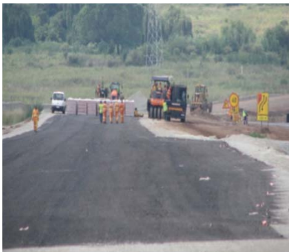
Voortrekker Road – Phase 1 under construction
