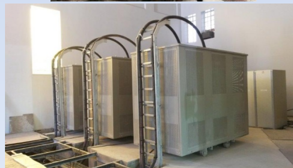
New variable speed drives
