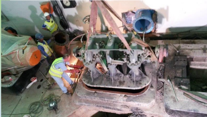
Old High lift pumps removed
