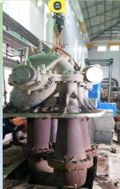
Old pumps and pipework removed
